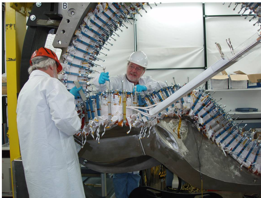
Figure 15: Modular coil winding operations at PPPL.
