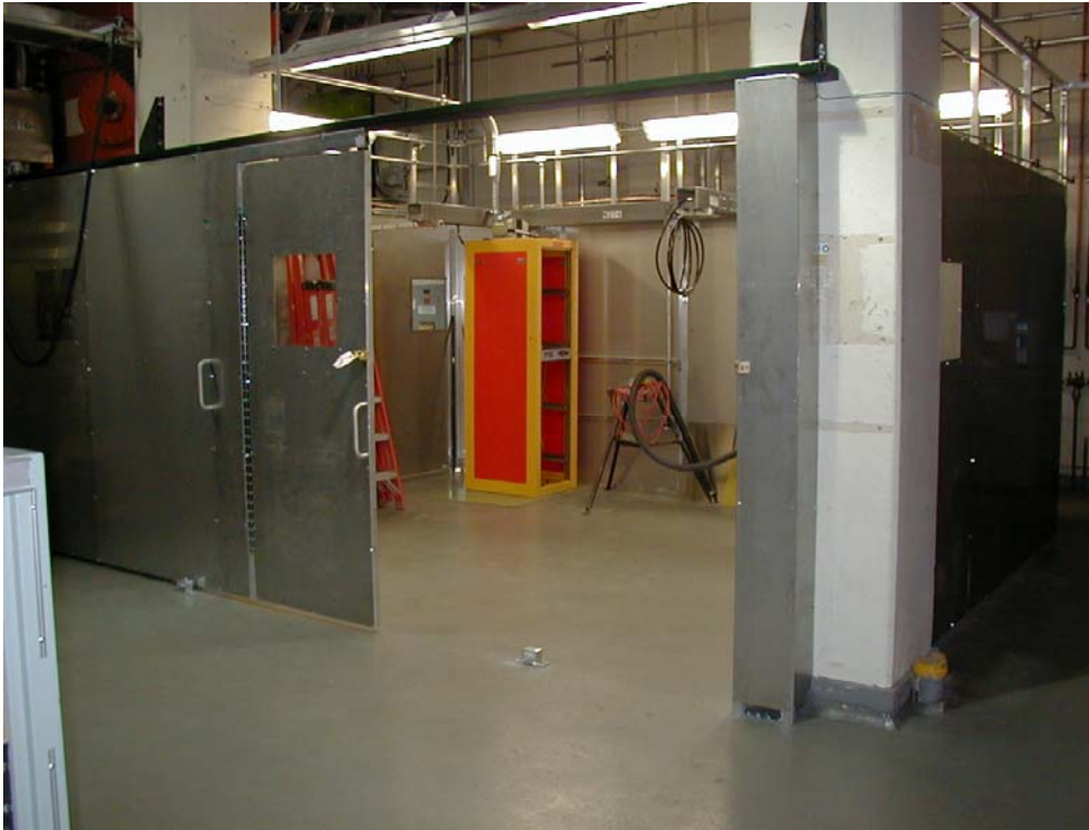
Figure 1 Coil Test Facility Enclosed Area
