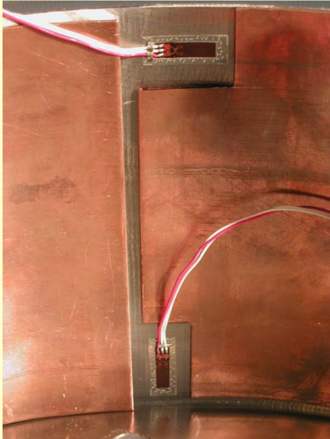
Fifteen strain gauges installed on winding form
