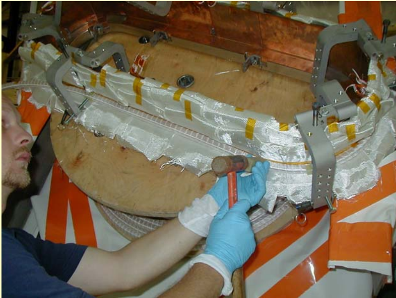
Forming conductor in place
