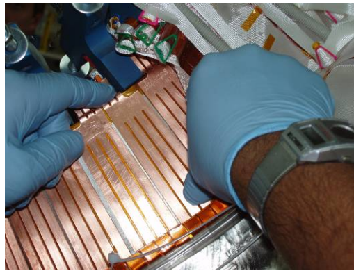
Figure 29- Positioning Vertical Cladding
