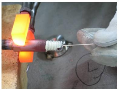
Figure 21- Feeding Sil-Fos Position C
