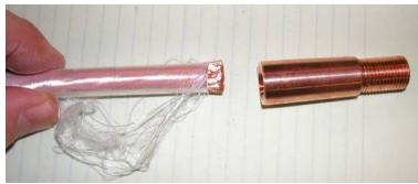
Figure 14- Removing Nylon Serve from Conductor
