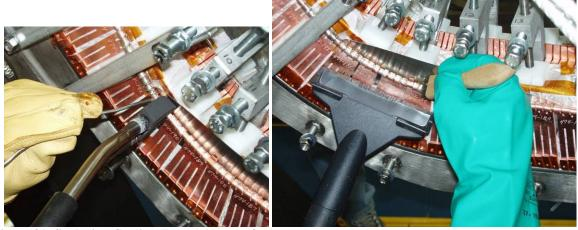
Figure 31- Soldering Cooling Tube (photos a & b)
