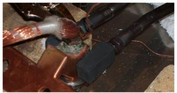
**Figure 43- Soldering Connector**
