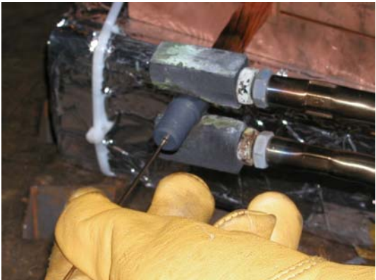
The Sil-Fos was fed through the feed-hole Figure 4
