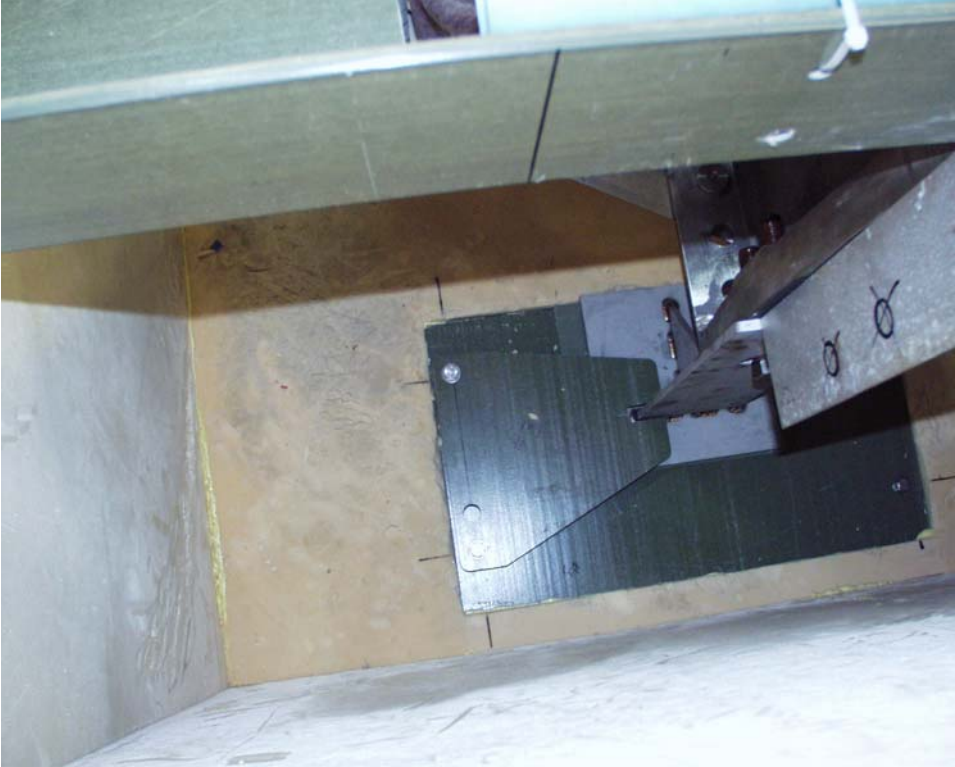
Figure 5-32 Restraints on C1 supports
