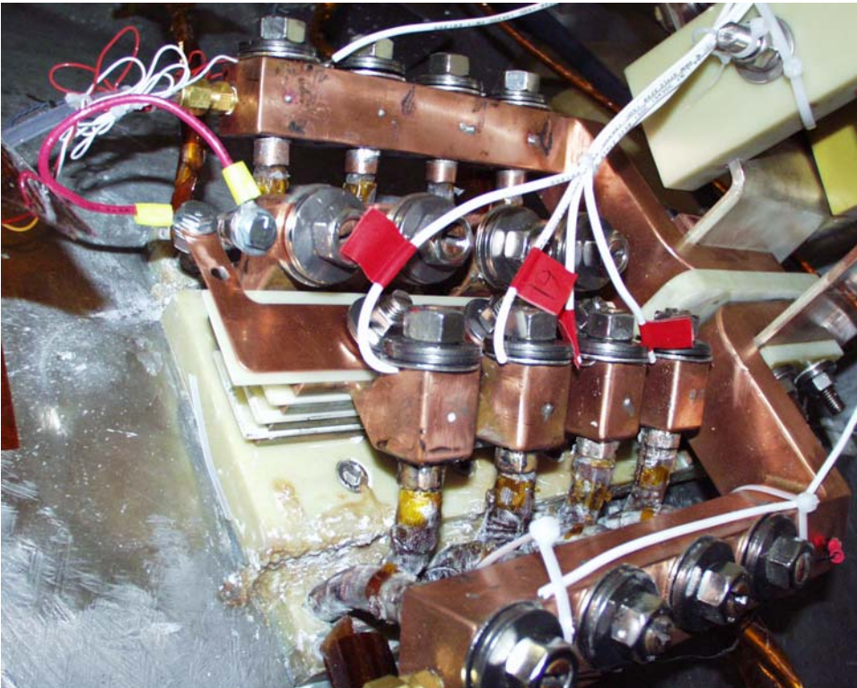
Figure 5-33 Instrumentation of jumper assembly
