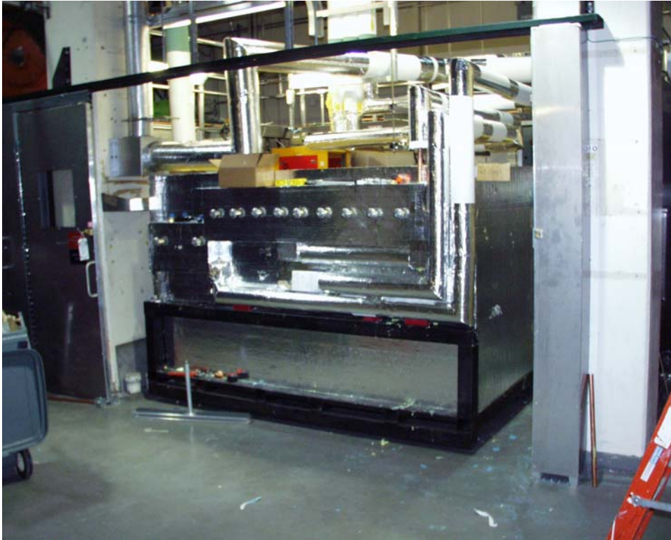
Figure 5-30 Cryostat inside Coil Test Facility
