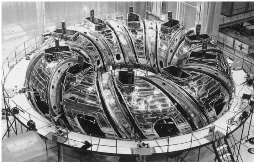
Fig. 7. Construction of the plasma vacuum vessel. Twenty half sector units of the vacuum vessel are installed between the helical coils on the winding core.
