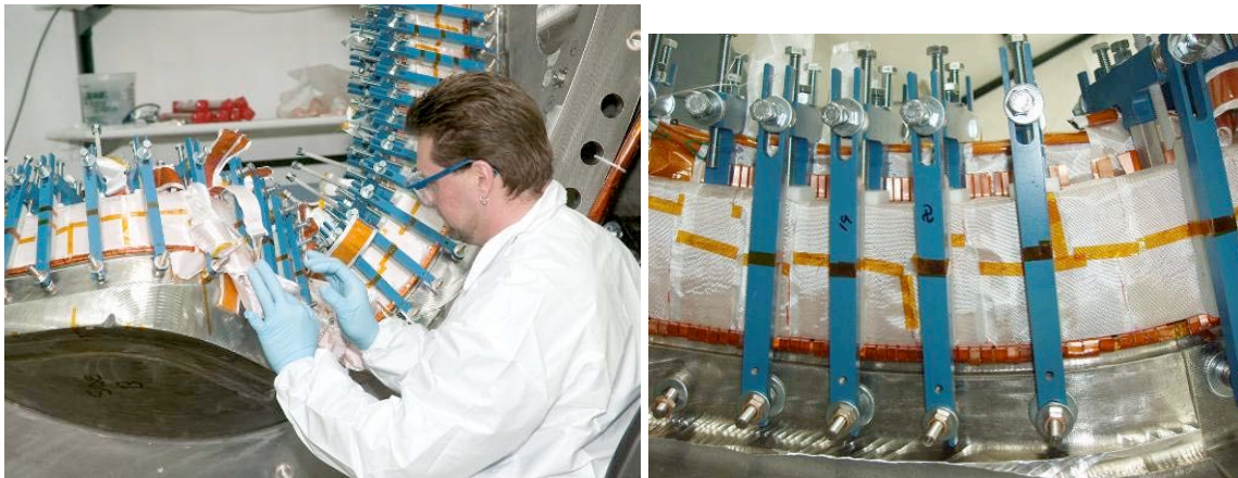
Finalizing the Groundwrap insulation
