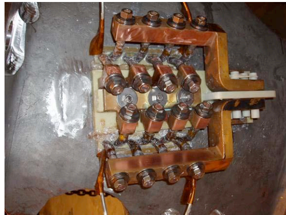
Modular Coil Lead Area
