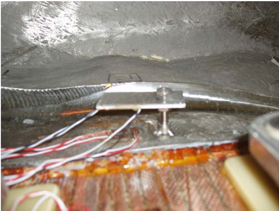
Figure 5-35 Casting strain gages at Clamp 68 - Side B
