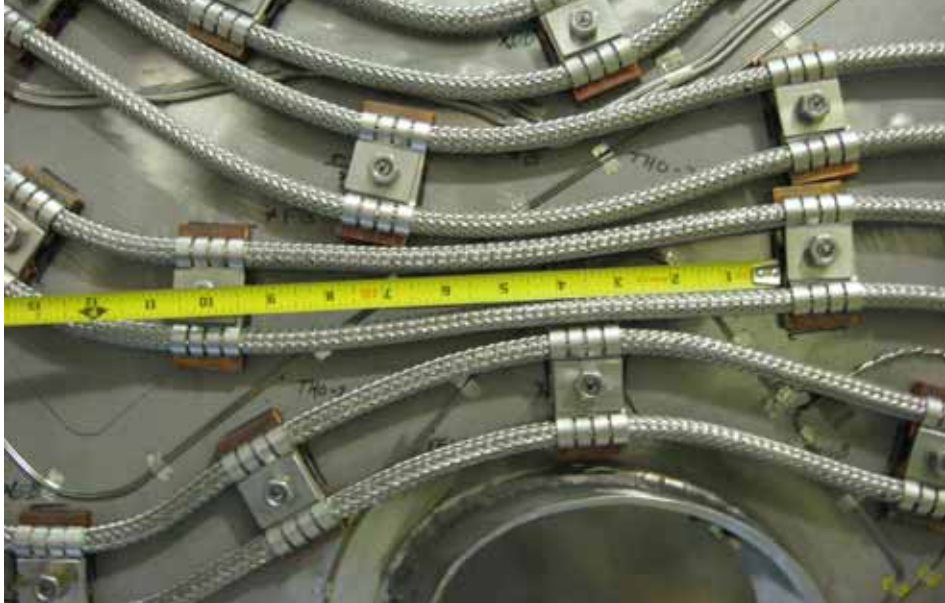
VVSA-3 - Spacing between H/C lines 9.5" near port 5A
