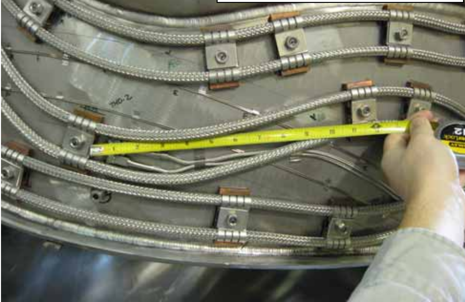
VVSA-3 - Spacing between H/C lines 11" near port 4B
