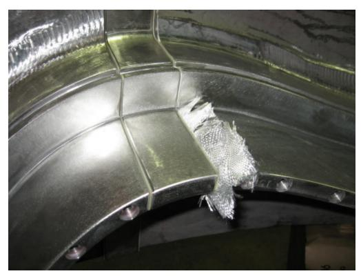
One side of the ¾" section of T accepted a .018" shim. The maximum allowable gap is .005". This area was repaired using fiberglass filler and now a .005" shim will not pass through this area.
