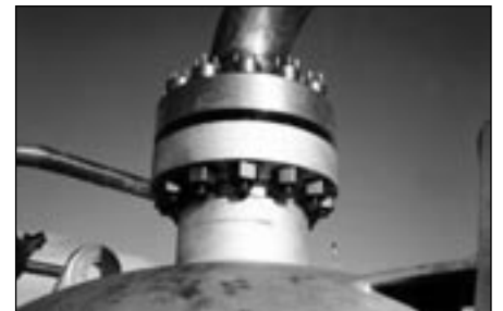
Severe temperature swings previously caused this flange to leak. Superbolt tensioners eliminated this problem. Also, because only hand tools are required, the worker can safely climb to this elevated worksite.
