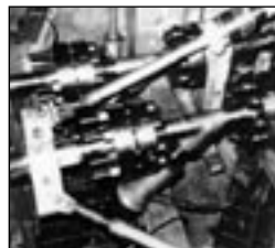
PORV - Pressurizer relief valve.
