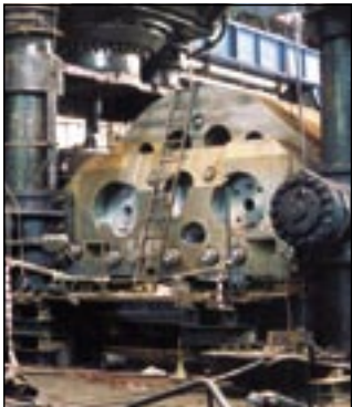
Press Platen repaired with tie bolts and Supernuts.
