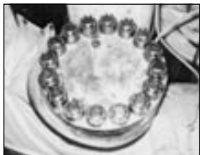
Pressurizer main steam safety valve.
