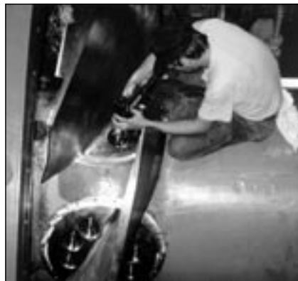
Armored Torquebolts used to secure blades on this hydro turbine.
