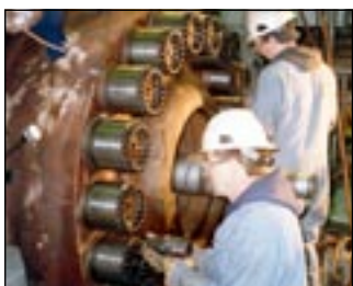
Two workers needed only 1 hour and 21 minutes to tighten these 5" tensioners.
