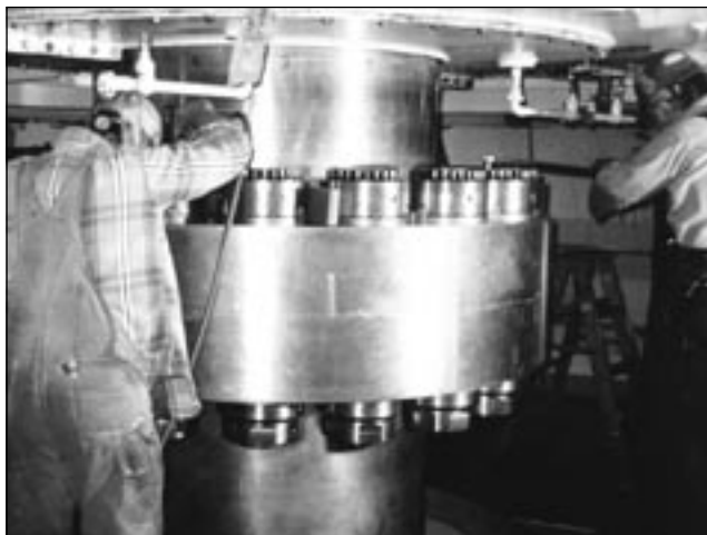
Kaplan Turbine Coupling, (18) 6-3/16" studs. The previous method required 150-250 man hours utilizing a 150 lb. "dead man", a 50 ton hydraulic ram, and a 250 lb. wrench. Supernuts® were installed in 2-1/2 hours using 1/2" air impacts and hand torque wrenches.
