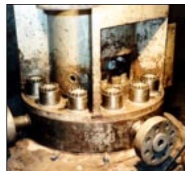
Superbolt tensioners make fast work for boiler circulating pump bolting.
