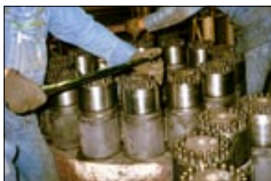
Outage time was reduced on this turbine stop valve.
