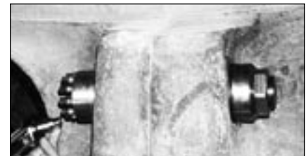
Split Gear segment on rotating kiln.
