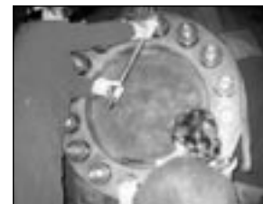
Severe temperature swings previously caused this flange to leak. Superbolt tensioners eliminated this problem. Also, because only hand tools are required, the worker can safely climb to this elevated worksite.
