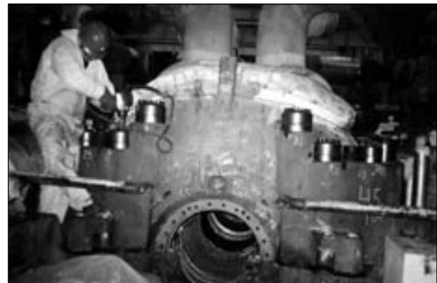
MT Supernuts® used as a closure tool. The shell had to be bolted up without the rotor assembly for measurements. The tensioners were used to speed up the maintenance schedule thus saving valuable outage time. Supernuts® are reusable for repairs on other turbines within this utility.
