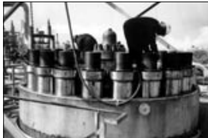
Large methanol reactor with 11" studs. Six hours with Superbolt vs. two days with Hydraulic Tensioners.
