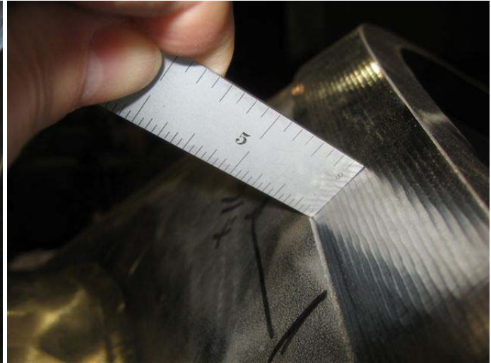
10 O’clock outside of Flange A
