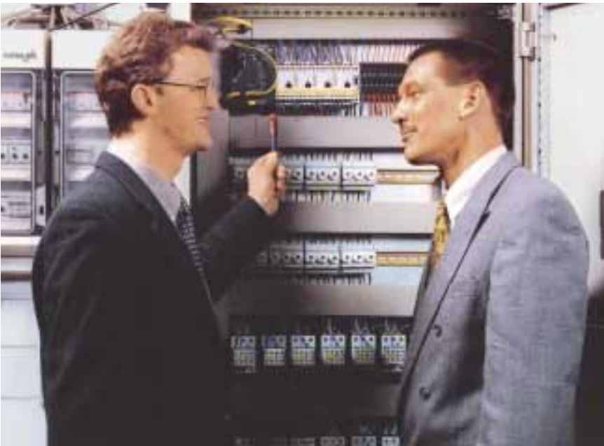
Stefan Höfer (right) Manager of the UPS Center Aachen and Heinz Czichy, Siemens consultant are very happy about the new and simple safety solution using AS-i Safety. As a result of the centrally located electrical cabinet, special AS-Interface cabling was able to be implemented
