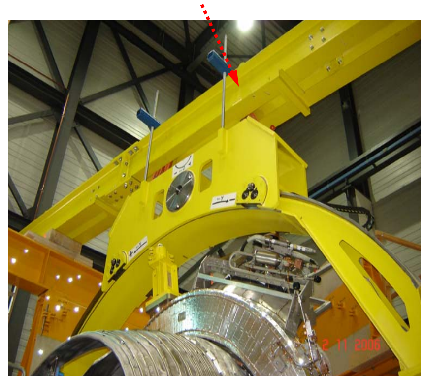
Figure 10: SAE-1 parking test without NPC3. The cross beam for coilparking is constructed by IMG, Rostock. Interaction between SAE-1, mobil crane, operating platform and headover crane.
