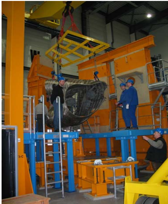
Figure 7: The cross beam for sector transport is constructed by DWE MAN.
