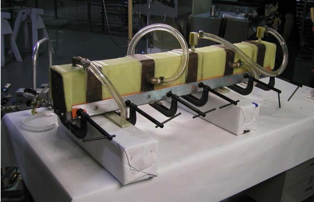
Installation of Outer Epoxy Shell (Strong back) is complete. Reinforcement bars placed on edge of mold to secure seams Figure 9
