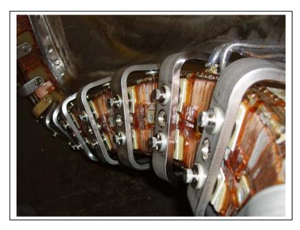
Original clamp arrangement can be used for majority of locations on the type C coils
