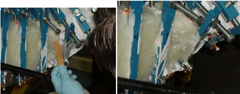
Figure 43-Application Epoxy Glass Shell
