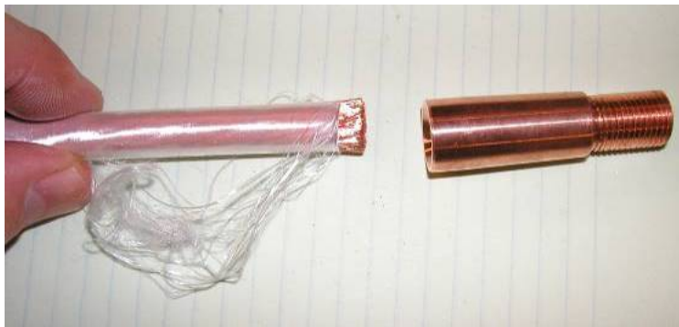
Figure 14- Removing Nylon Serve from Conductor
