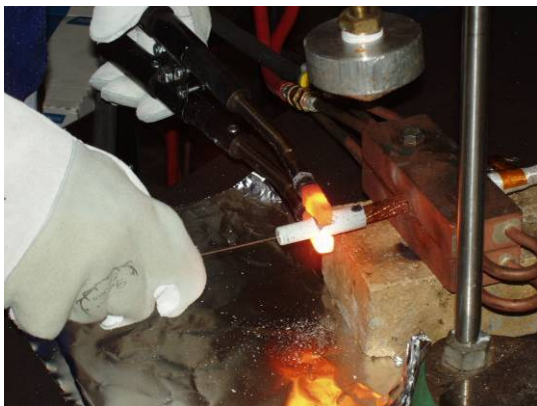
Brazing Copper Lugs onto Conductor
