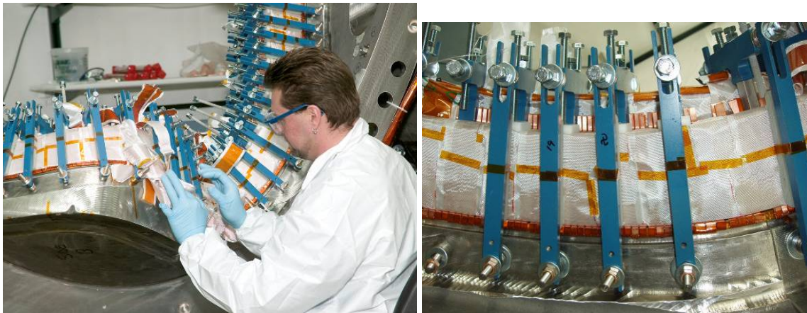
Finalizing the Groundwrap insulation
