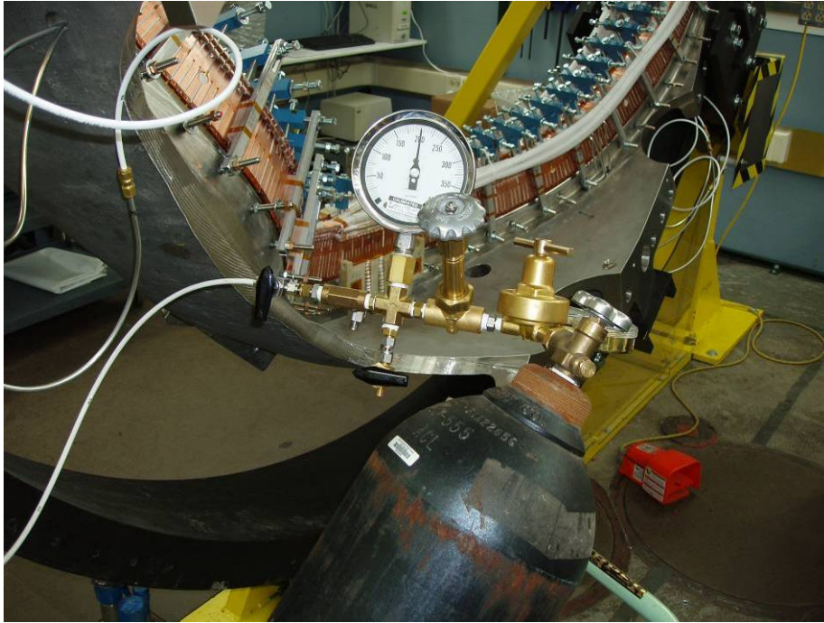
Pneumatic Test Setup for checking cooling tube system
