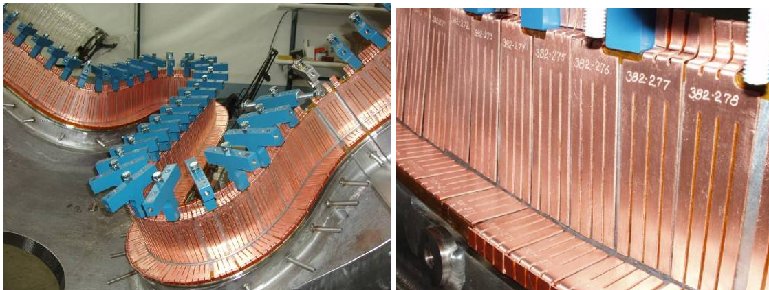
Copper Cladding Installed
