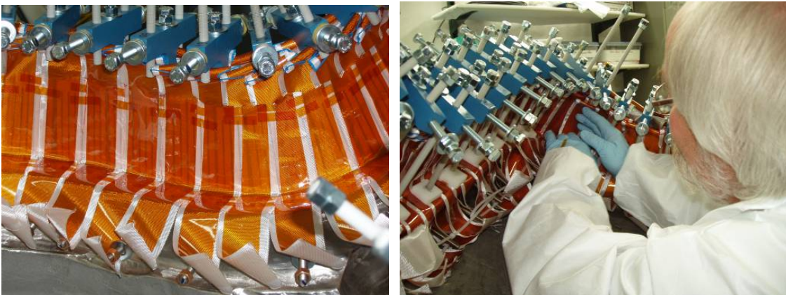
Applying Ground wrap insulation
