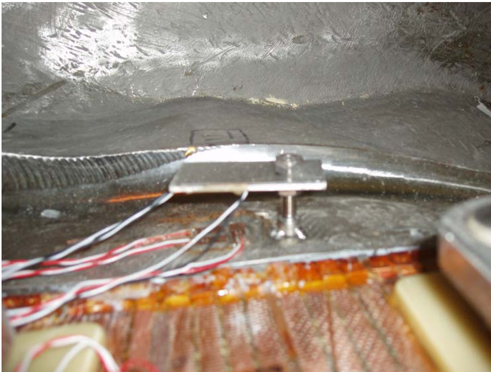
Figure 5-35 Casting strain gages at Clamp 68 - Side B
