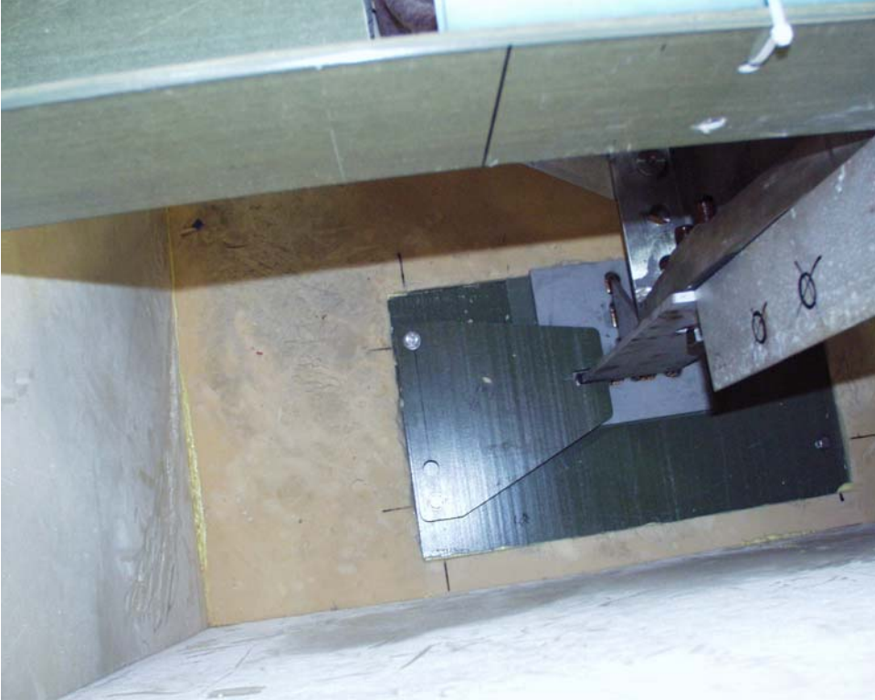
Figure 5-32 Restraints on C1 supports
