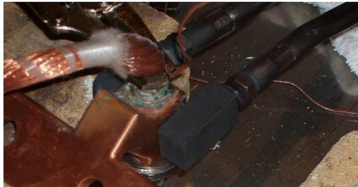
Figure 43- Soldering Connector
