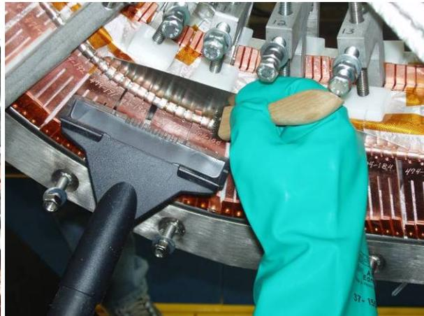
**Figure 31- Soldering Cooling Tube (photos a & b)**
